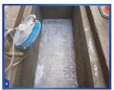
Especially in the closed areas it will be useful to make air circulation by a fan and to accelerate the drying by an electric heater. For the decorative viewed pools, blue color Molumer Pool Paint can be applied.
